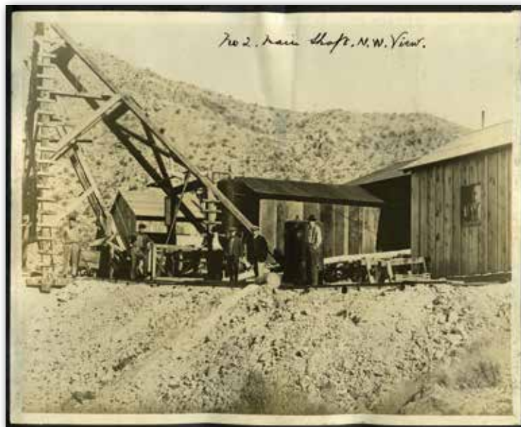
Figure 12. View from the northwest with five men posed adjacent to the A-frame, mine shaft and engine house building at the No. 2 main shaft. Operations at the mine opened and closed as market prices changed. Despite the No. 1 shaft being deepened to 225 feet, it soon became clear that the ore was not rich enough to support productive commercial mining operations, given the high cost of transporting the ore. Security threats during the 1920s also limited mining. (Silver print, photographer unknown, ca 1920s.)
