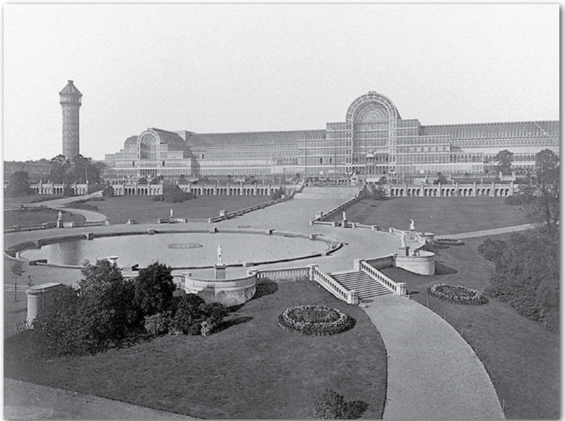
Figure 3. The "Crystal Palace" photographed with the view from the Water Temple taken by Philip Henry Delamotte, January 1, 1854. [Author's collection]
